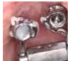
Only when “spaghetti” exits from the holes of the collar on the side is it completely filled.
